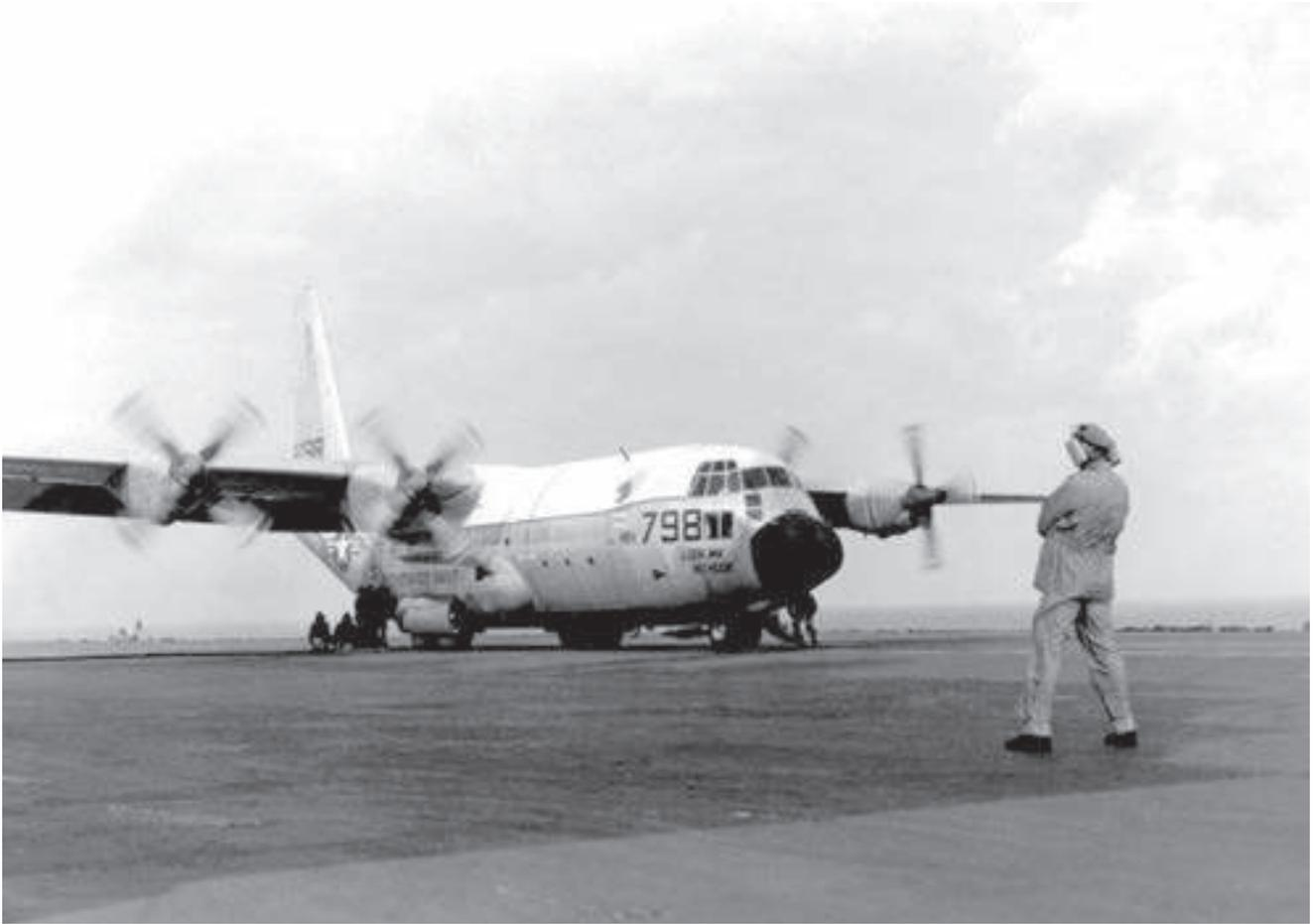
*In addition to testing the basic feasibility of landing a Hercules on an aircraft carrier, the project was also designed to make landings at increasingly heavier weights to determine how large a payload a C-130 might safely bring aboard. Because the aircraft was a tanker, simply adding additional fuel increased the gross weight of the aircraft. Here, the deck crew adds fuel to the KC-130's fuselage tank*
